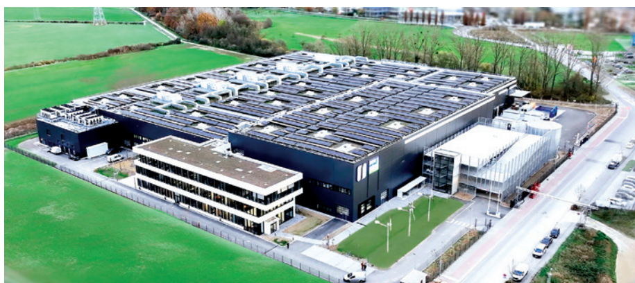
Figure 1: Sustainability measures can include installing solar panels and wind turbines at manufacturing sites.
